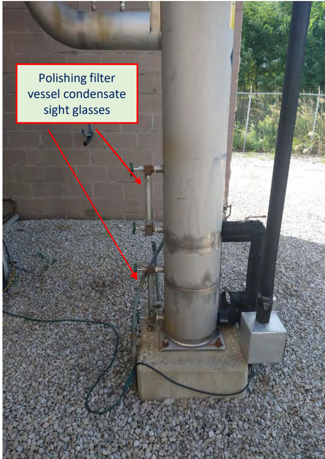
10. Polishing filter vessel condensate sight glasses.
