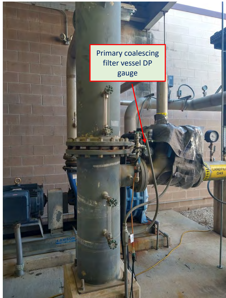
5. Primary coalescing filter vessel DP Gauge
