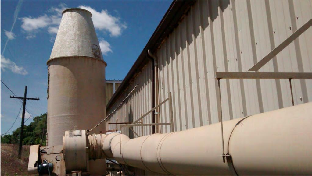
Photo 1: View of scrubber for the nickel plating process and its ductwork, and the south exterior wall (2016).
