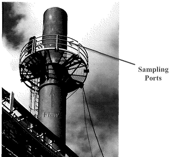
**Figure 2-3. Boiler No. 5 (EUBR05) Exhaust Stack**
