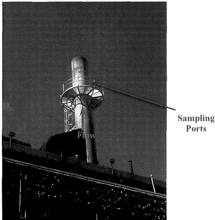
**Figure 2-2. Boiler No. 3 (EUBR03) Exhaust Stack**
