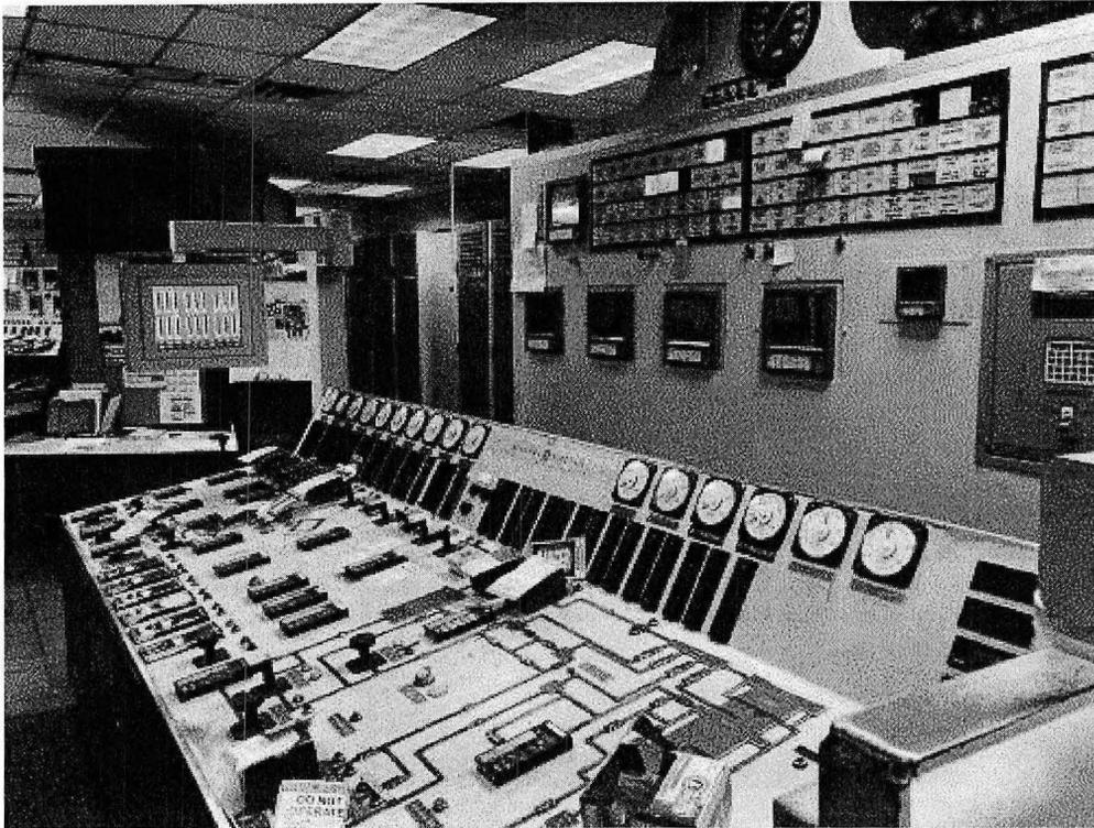
Image 3(056) : Locked Out/Tagged control room at Eckert Station
