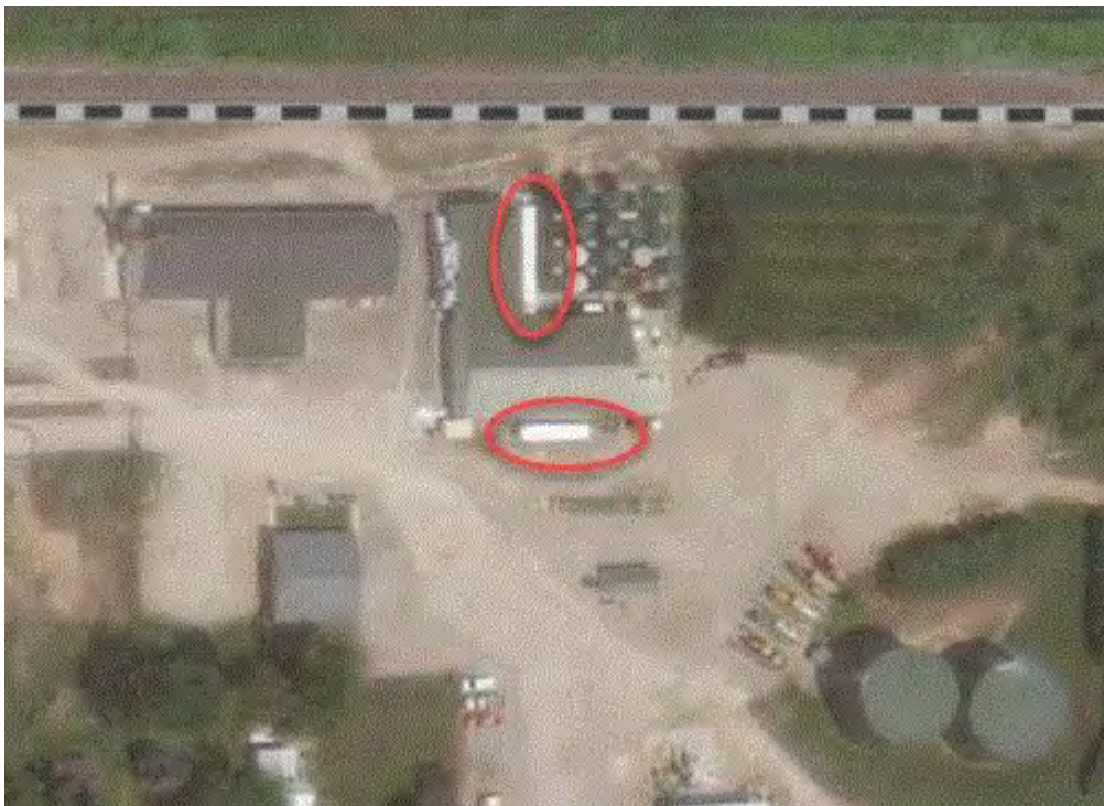
Image 1(NH3 tanks installed) : Aerial Bing maps photo of the site prior to removal of the 2 tanks.
