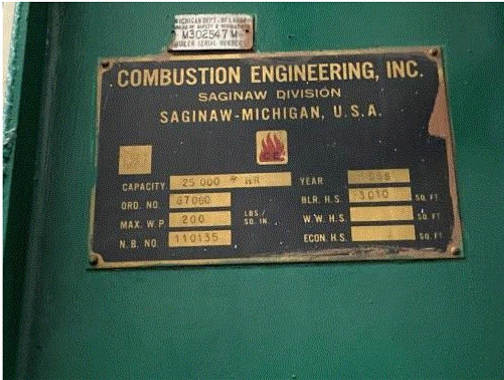
Image 2(1969 Boiler Plate) : Boiler plate
