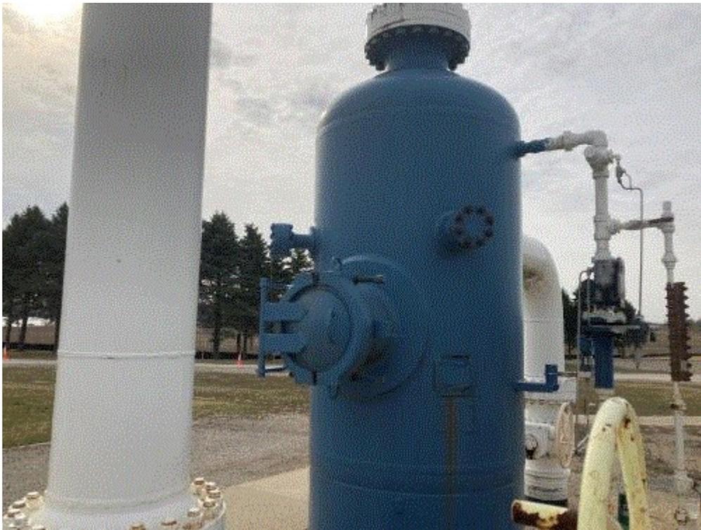
**Image 3(Suction scrubber)** : Suction scrubber leak..east tank.
