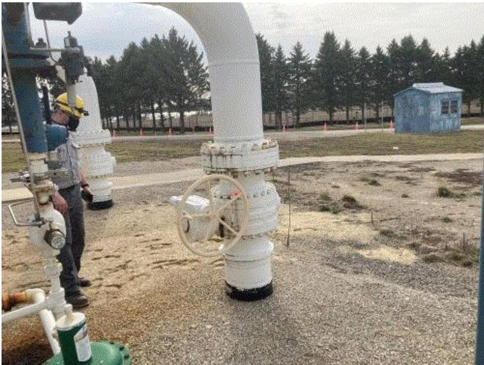
**Image 5(Suction scrubberpipe)** : Behind west suction scrubber.....pipe leak.
