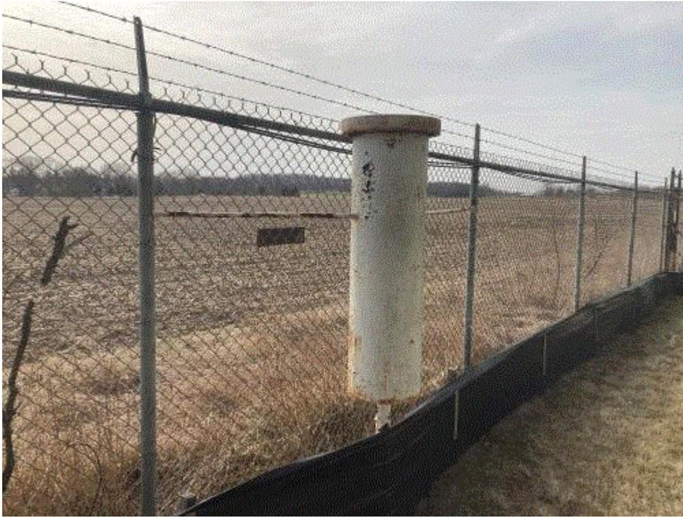
**Image 8(Plant 2 blow down)** : Vent pipe associated with plant 2 blow down
