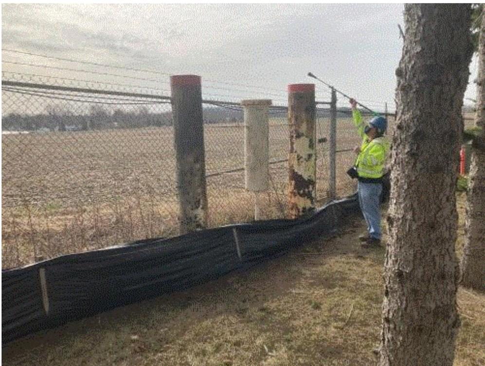
**Image 7(Plant 1 blowdown) :** 3 blowdown vents associated with Plant 1 that had methane emissions.
