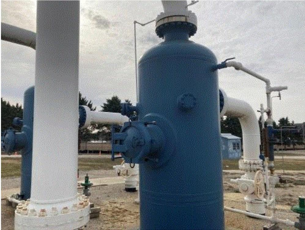
**Image 4(suction scrubber)** : Suction scrubber leak-west tank.
