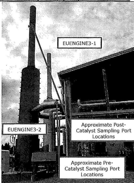
**Figure 4-2. Post-Catalyst Sampling Port Location**
