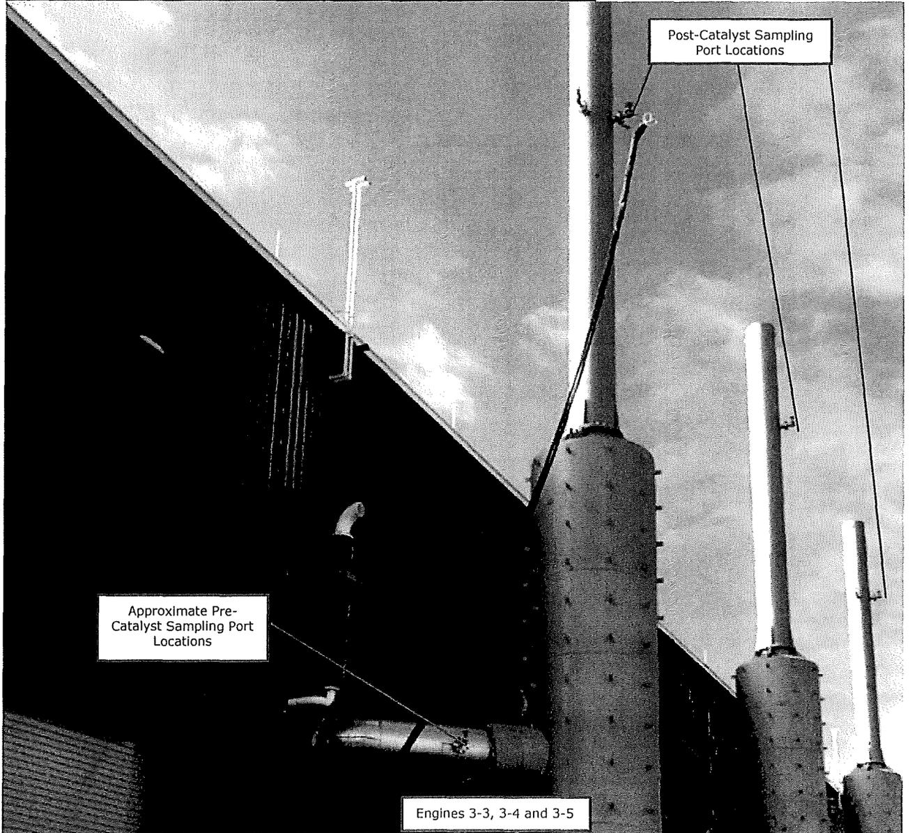
**Figure 4-2. Post-Catalyst Sampling Port Location**
