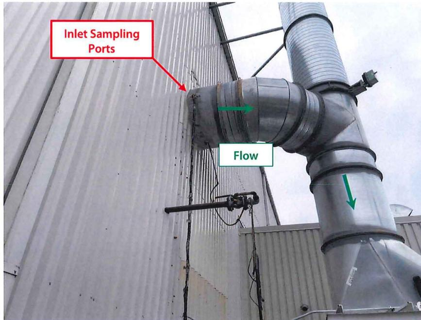
**Figure 2-1. RTO Inlet Sampling Location**
