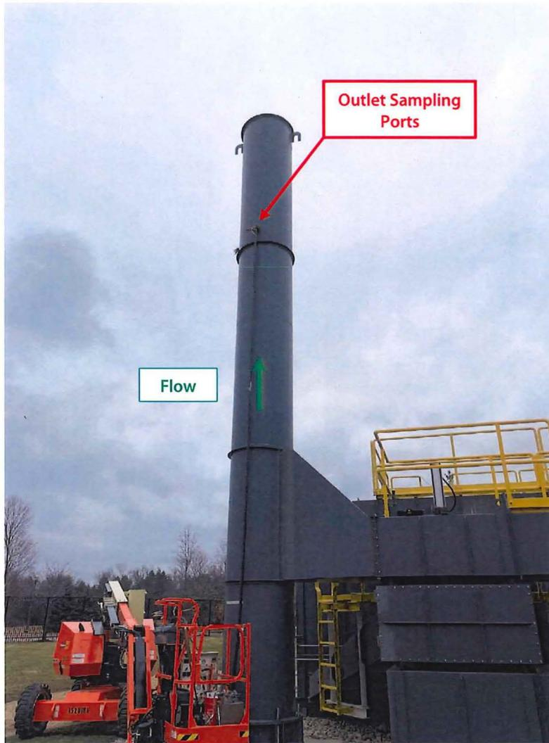
**Figure 2-2. RTO Outlet Sampling Location**
